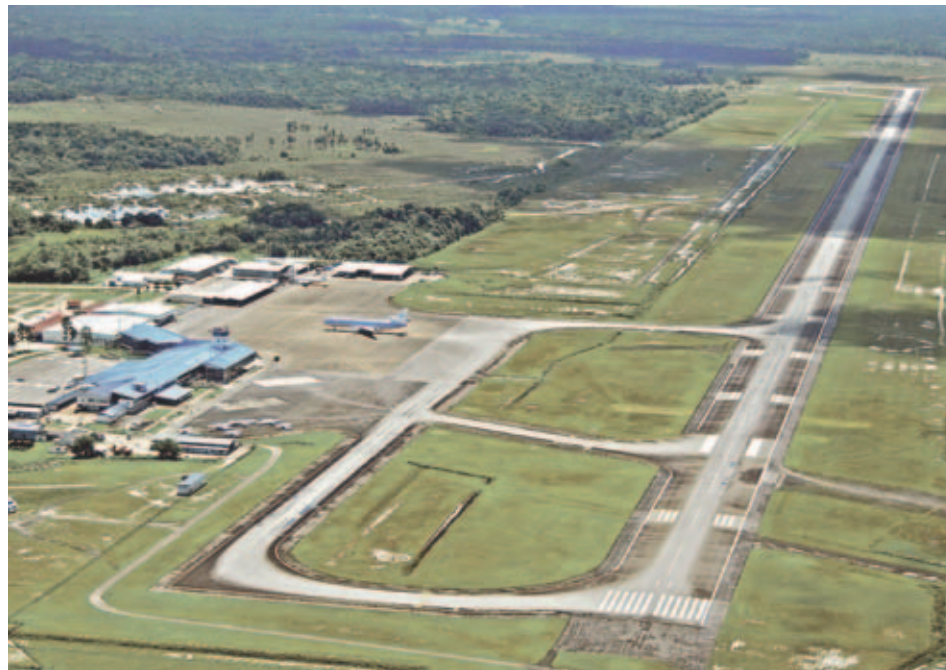
N.V. Luchthavenbeheer has carried out asphalt projects at the capital's Johan Adolf Pengel International Airport (JAP) Airport
